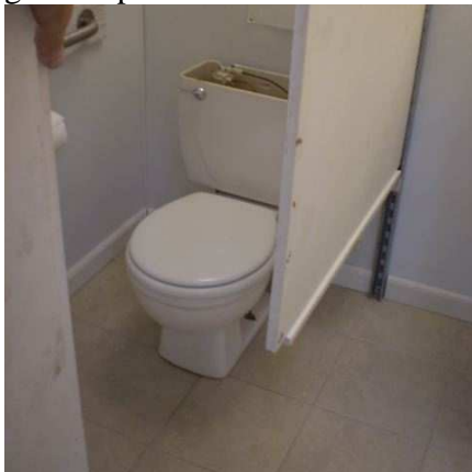
Floor Tile, FRP Walls, and Partitions in Men's Room
