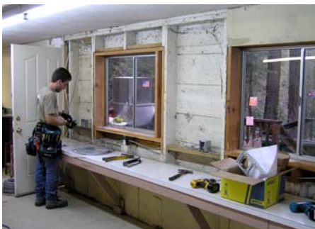
Mike Hulbert wiring electrical boxes
