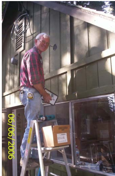
Rich Holden installing new light fixture on front of dining hall
