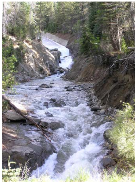
Below the Bucks Lake spillway in early June (usually dry in the summer)
